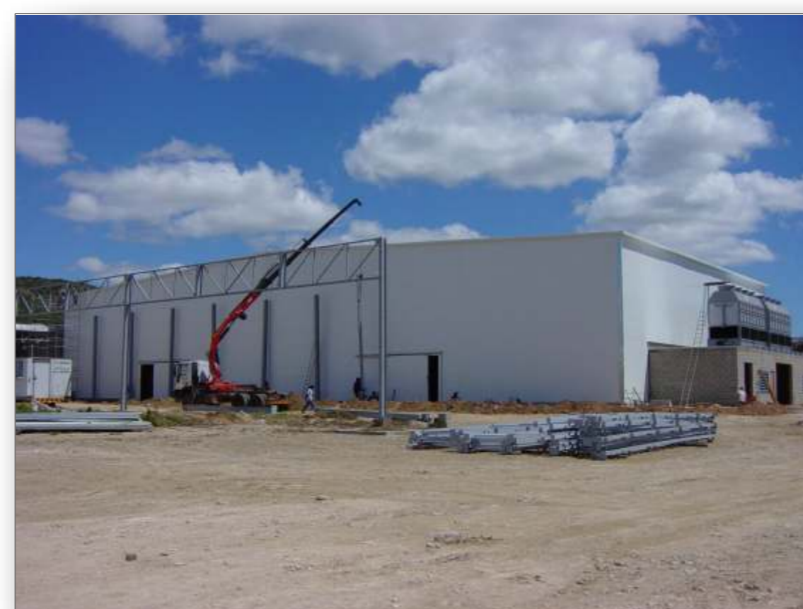
Apple Storage facility for Unifrutti
