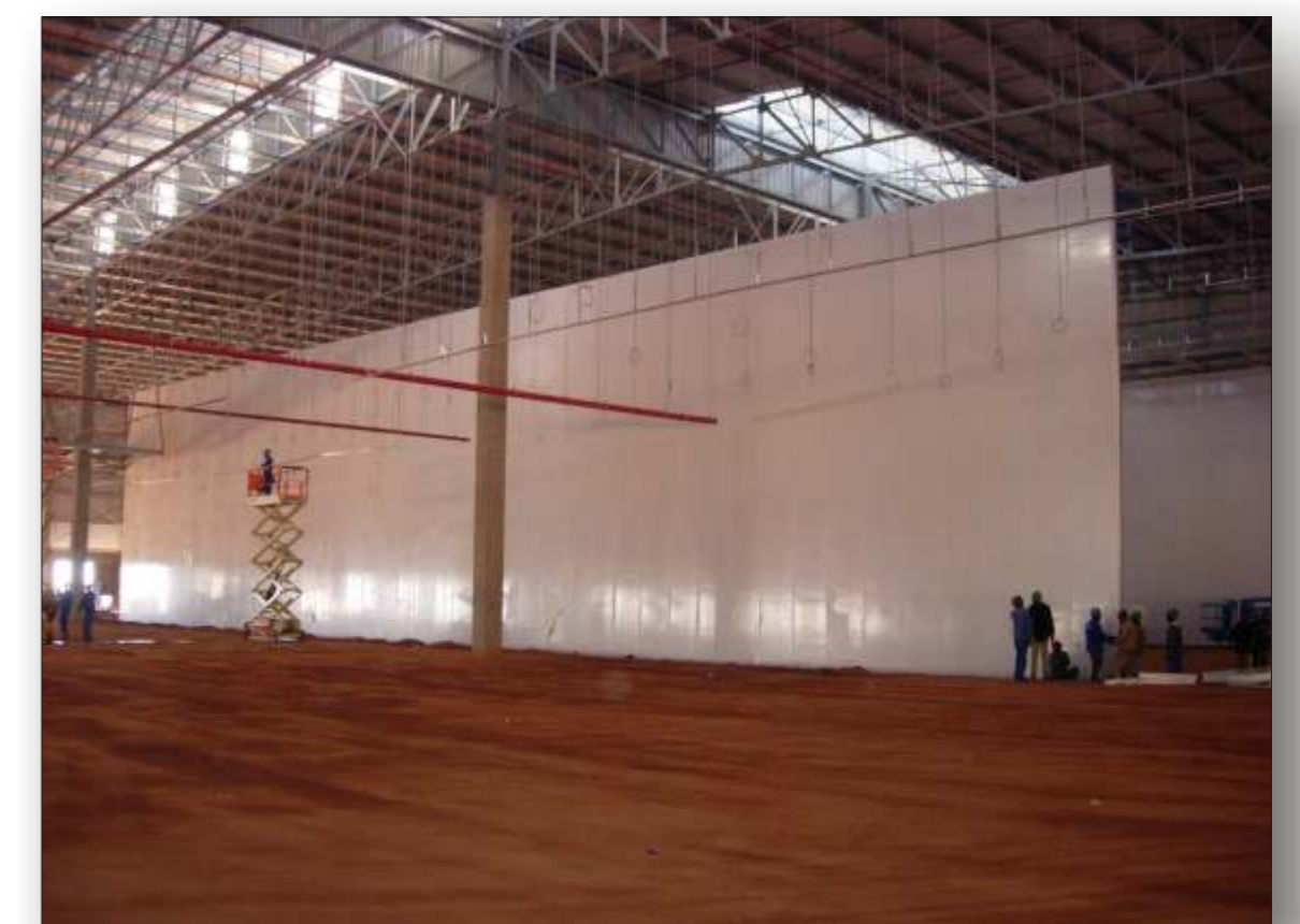
Woolworths Freezer Distribution Centre under construction
